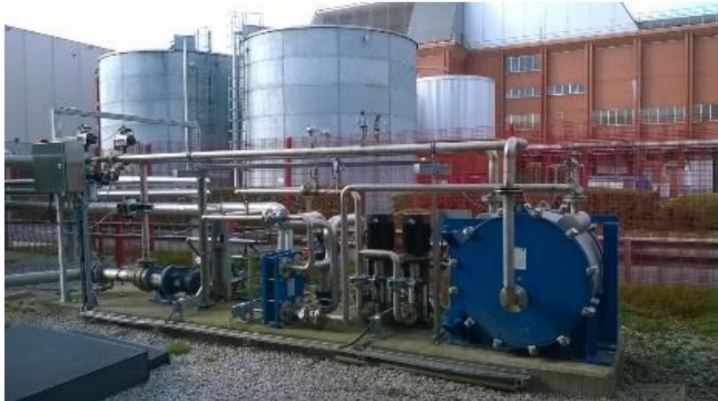
minimising blockages. The spiral heat exchanger is designed specifically for high solid rates, such as pulp and sludge, and an automated backwash system maximises the availability of heat recovery to the site.
